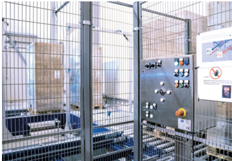
Two control cabinets are used for manual control. These contain FEN20 multiprotocol modules, which expand the number of inputs and outputs available
