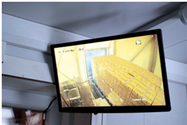
The driver presses a button to start the fully automated conveying of the pallets from the ATL zone to the refrigerated truck
