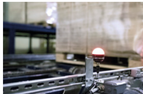
K50 LED lights from Banner Engineering provide important information about the status of the line modules
