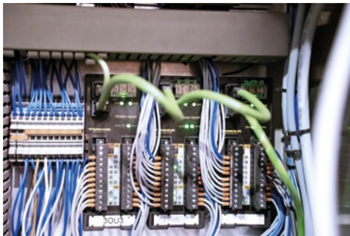
Turck's FEN20 devices make the switching signals of the control consoles bus-capable
