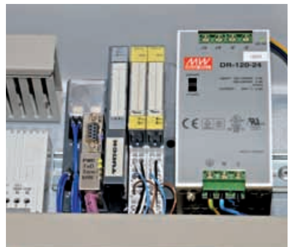
Four TI-BL20-DPV1 Profibus gateways transfer the RFID data to the database
